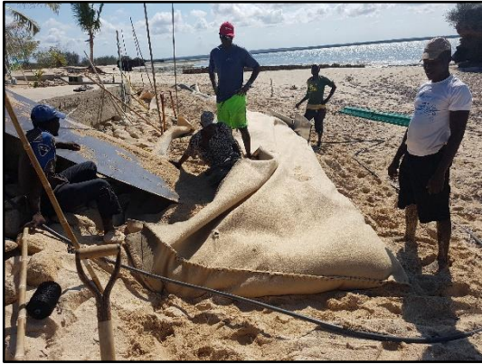
sewing the back closed
