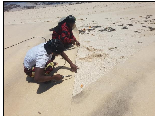
making holes for stitching
