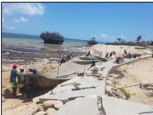
Placing of EnviroRock 3PL in position
