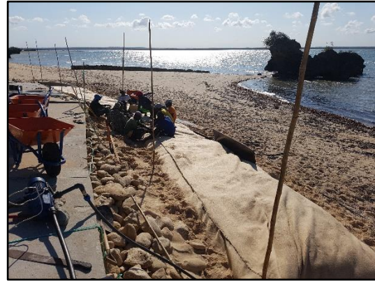
Sewing edges and filling corners
