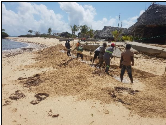
Excavation of foundation
